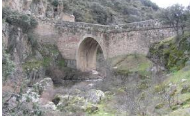
Cultural heritage restoration and preservation
